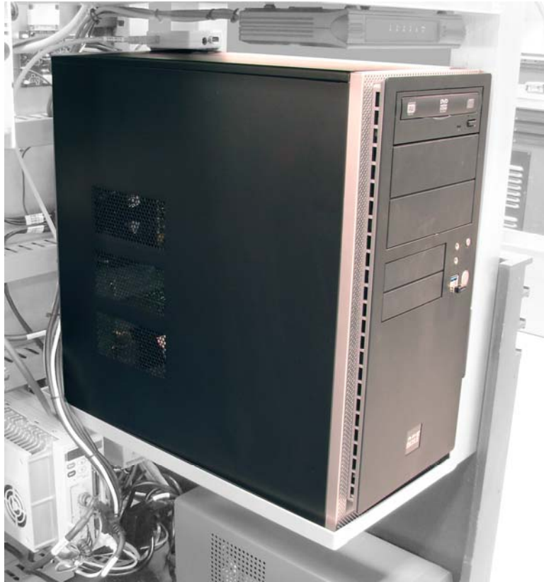
Shown in place
